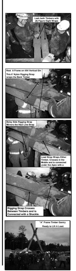
Erecting the "A" Frame
